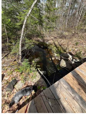
Sm. Bridge over Brook
